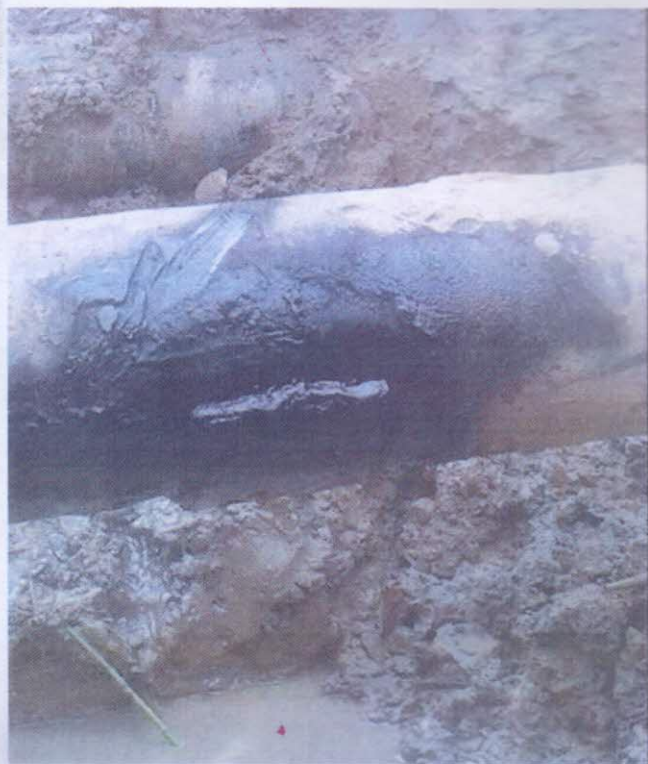
Figure 2: Weld part on the pipeline.
